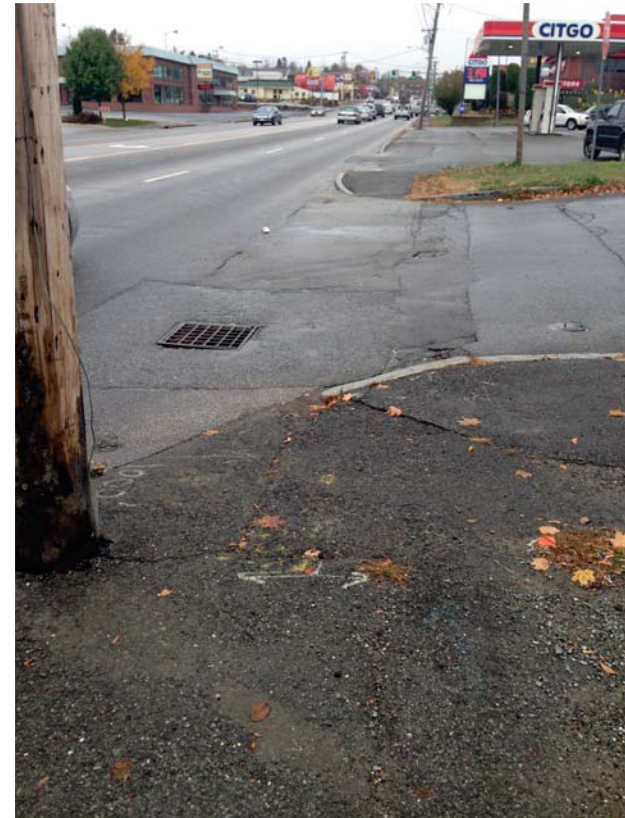
Figure: Poor curb cut, obstruction, restriping needed
