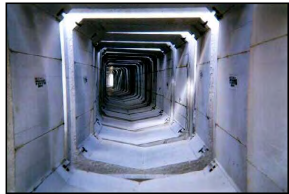
STOCKPILED PRE-CAST UNITS INSIDE VIEW
