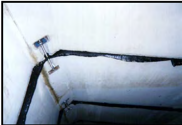
BOLTED JOINT CONNECTION
