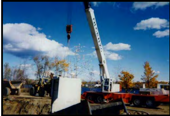
INSTALLATION OF NEW SECTION
