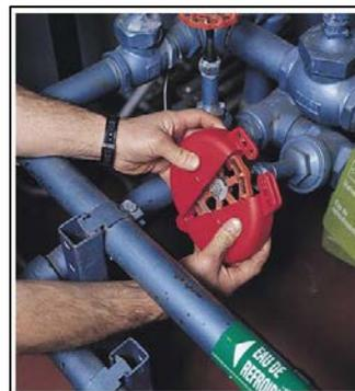
Valve Lockout Device
