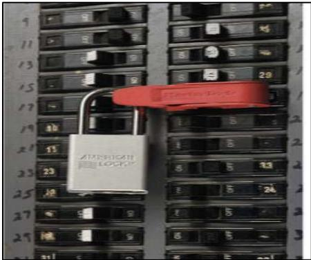
Circuit Breaker Lockout Device
