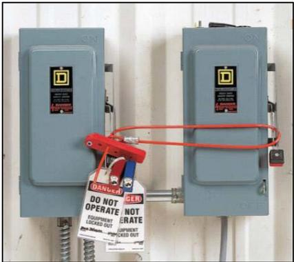
Cable Lockout Device
