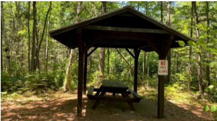
Example of covered picnic table site along the East-West Loop Trail near the Kittredge Road parking area
