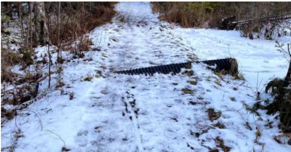
Example of a culvert on the East-West Loop Trail in December 2020
