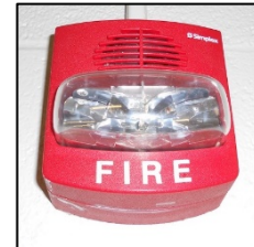
Fire Alarm Strobe Light
