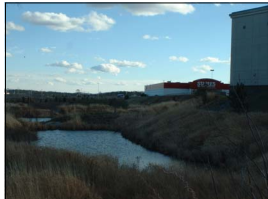
December 2004: Detention ponds and other BMPs can help reduce the impacts of impervious cover.
